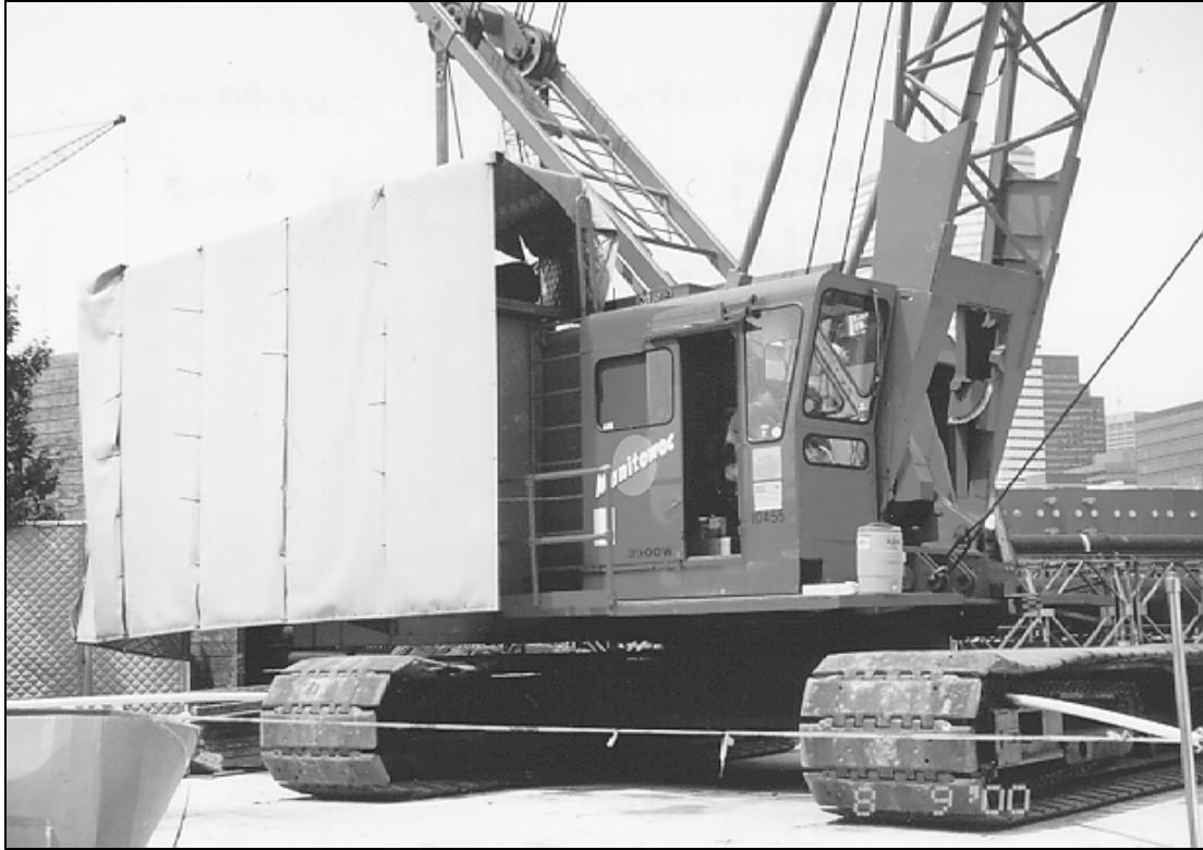
FIG. 3. Crane with noise curtains enclosing the engine and muffler area.
