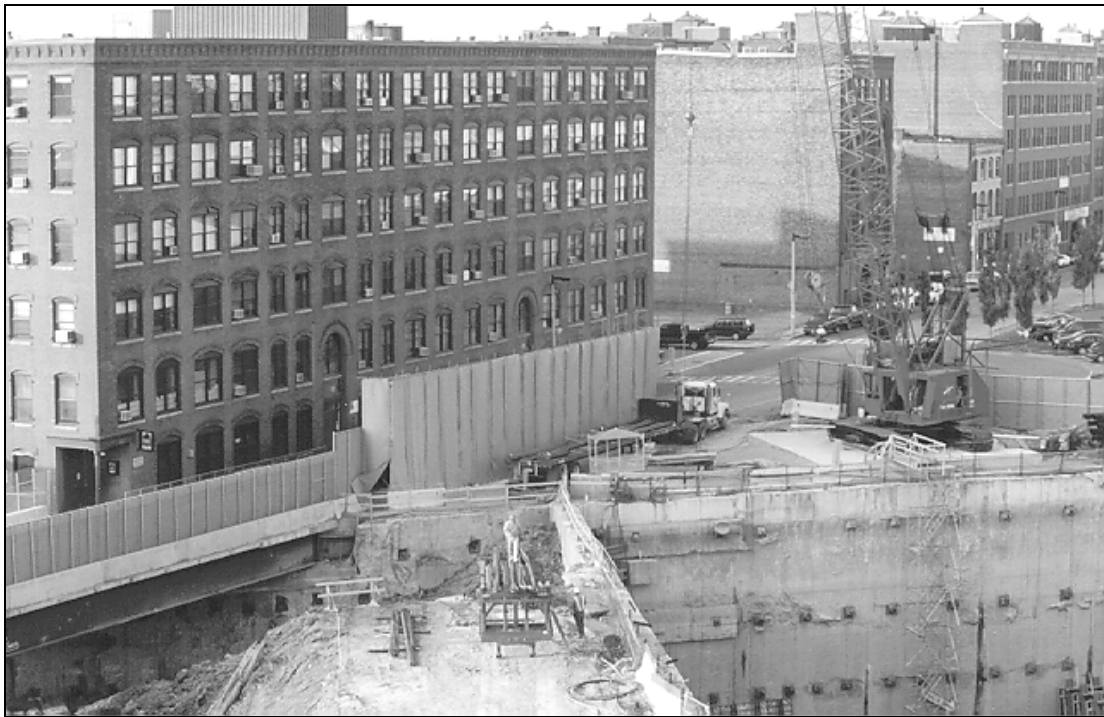
FIG. 2. Twenty foot tall noise barrier of scaffolding and noise curtains.
