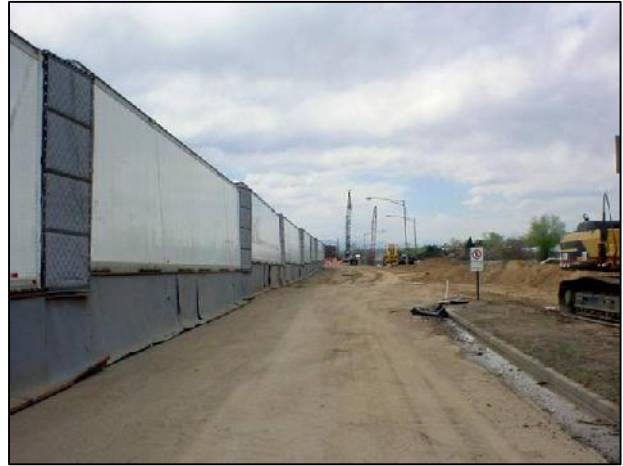
Photo 2. Trailers as Noise Barrier
