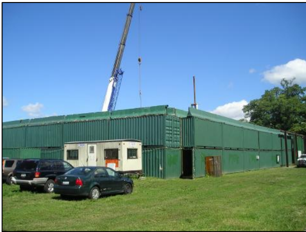
Photo 5. Conex Boxes as Noise Barrier
