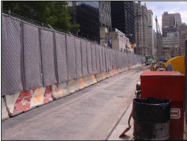
Photo 1. Plywood Barriers on Jersey Bases
